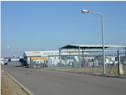
Figure 2.5 View south along Wackett Street to Sbell fuel depot (Building 655).
